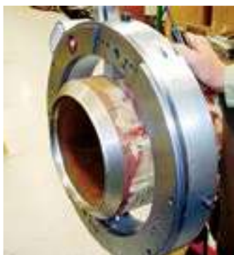
Weld ready after machining
